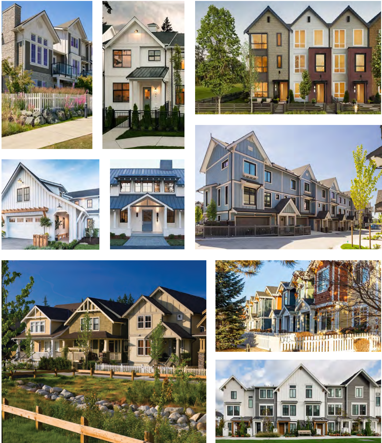
Figure 17: Neighbourhood Character | Residential – Ground Oriented
