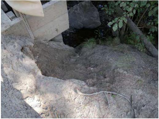
Photo 8: Erosion associated with a stream crossing.
