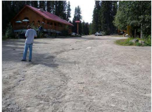
Photo 6: Moderate erosion associated with the boat launch at the Beaver Lake Lodge.
