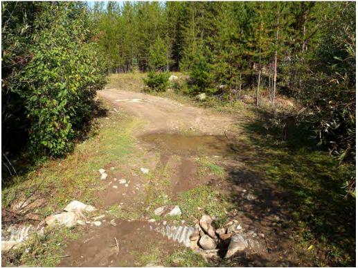
Photo 20: Example of a damaged culvert.
