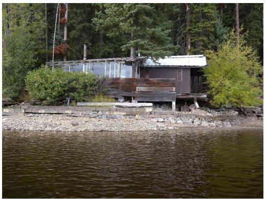
Photo 18: Example of a lease lot retaining wall likely constructed to prevent erosion.
