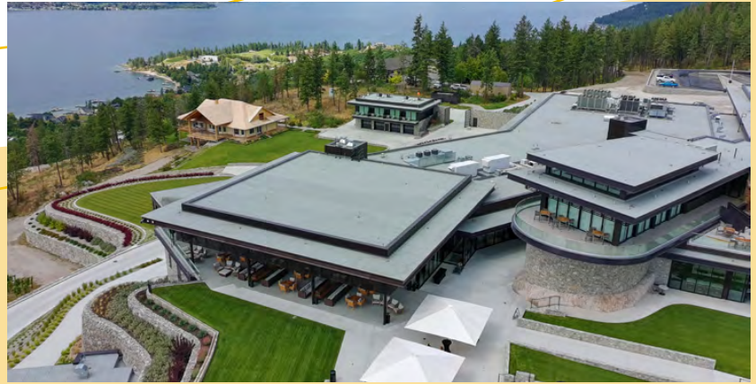
O'Rourke Family Estate Winery – vineyard, winery, restaurants, outdoor amphitheatre, and on-site accommodation (future event centre still under construction).
