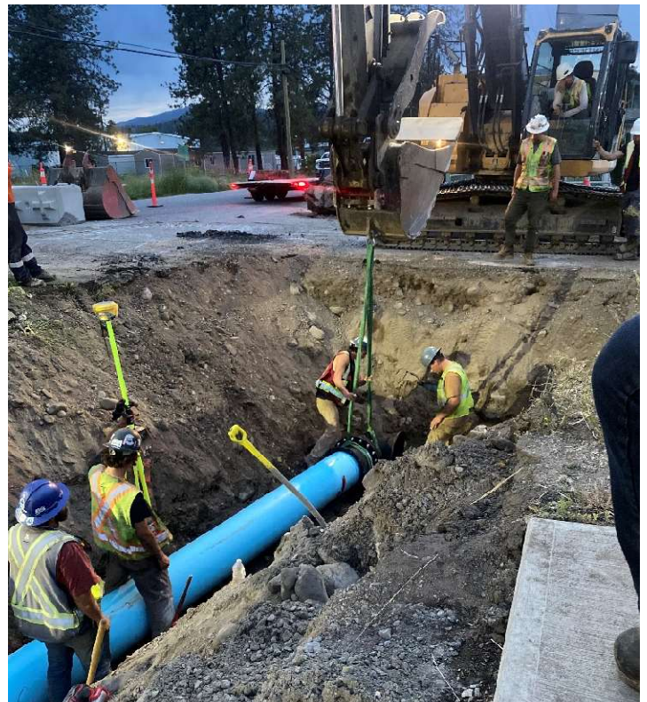
Figure 3 June 11, 2025, Water Main Tie-in Bulk Water Meter Project
