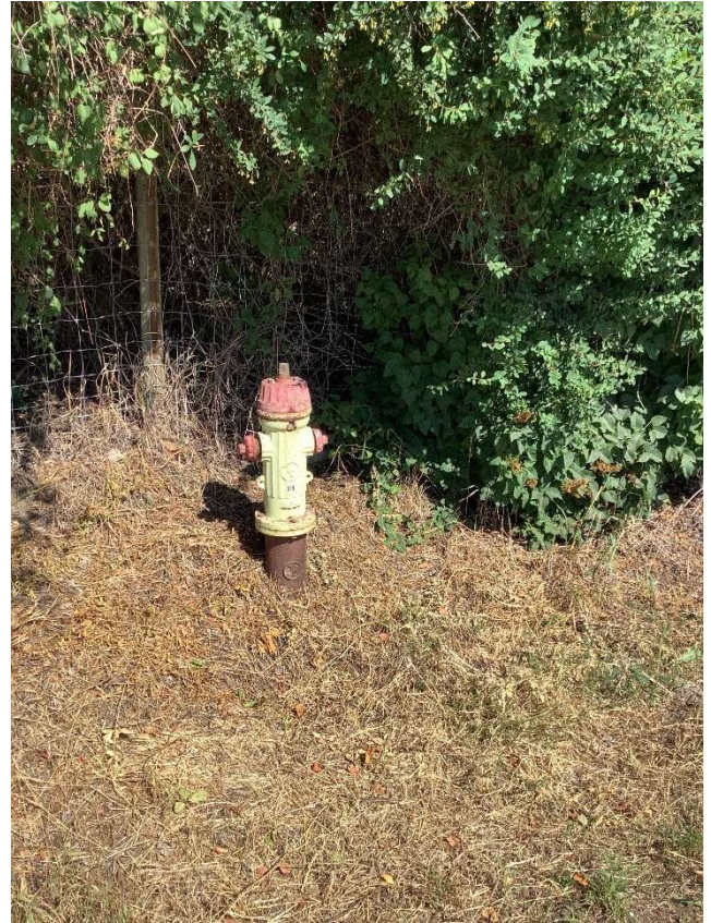
Figure 4 District of Lake Country Hydrant in Oyama
