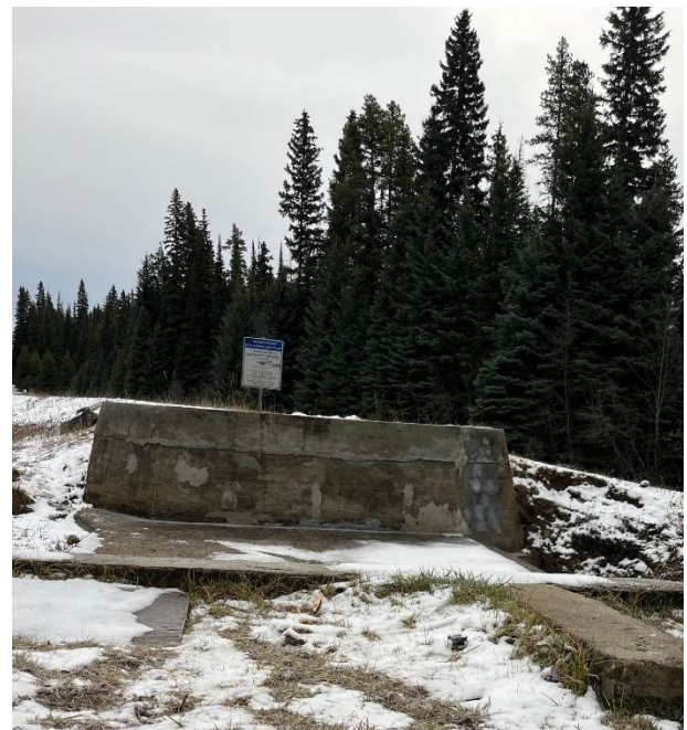
Figure 14 Crooked Lake Spillway
