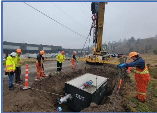
Figure 3: Installation of the vault housing the meter for the discharge to the City of Kelowna Collection System.
