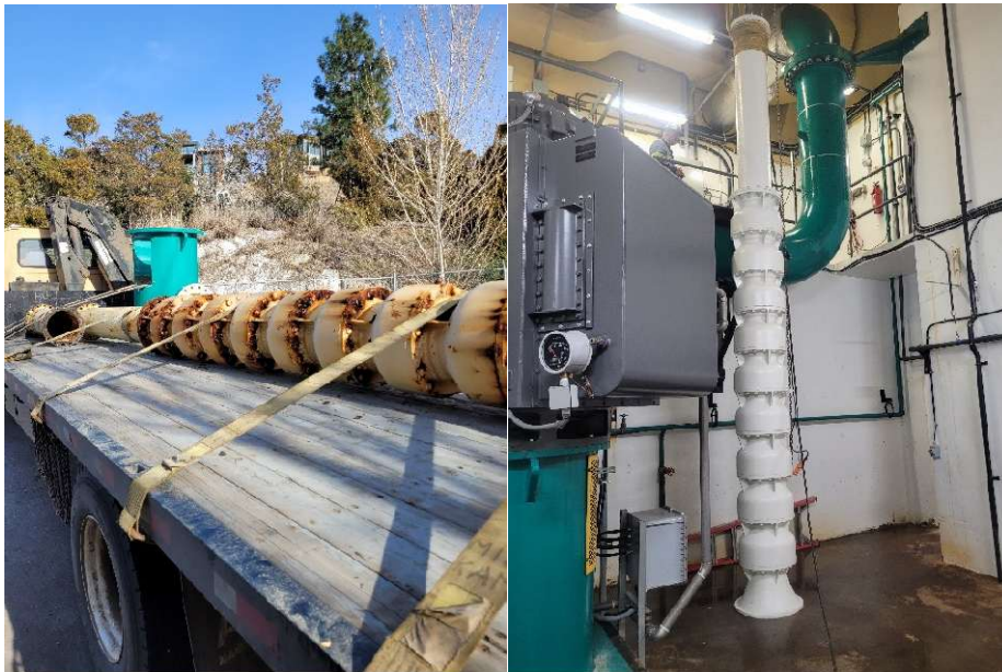
Okanagan Lake Pumphouse, pump installation
