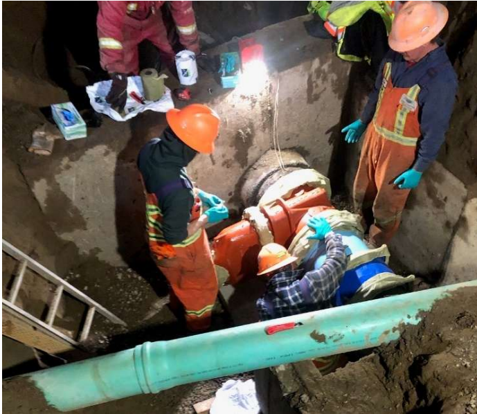
Installation of the new main line valve (left) and the shutdown area (right).
