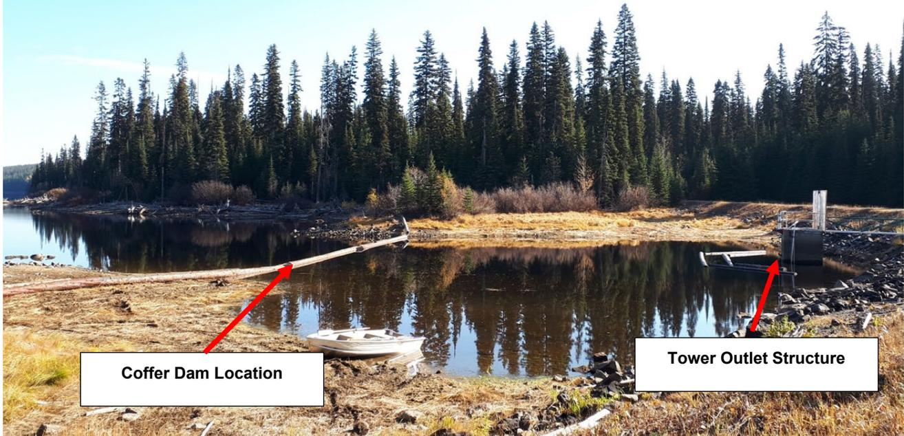
The Beaver Lake Dam's tower outlet structure is responsible for controlling water releases from Beaver Lake into Upper Vernon Creek. This structure has been identified as needing replacement. The last improvements to the structure were carried out in the 1980s. In 2017, a review of the tower revealed structural concerns, indicating that significant improvements, or complete replacement were necessary. A scoping report was finalized in 2019, and the multi-year design works were initiated in 2020.
