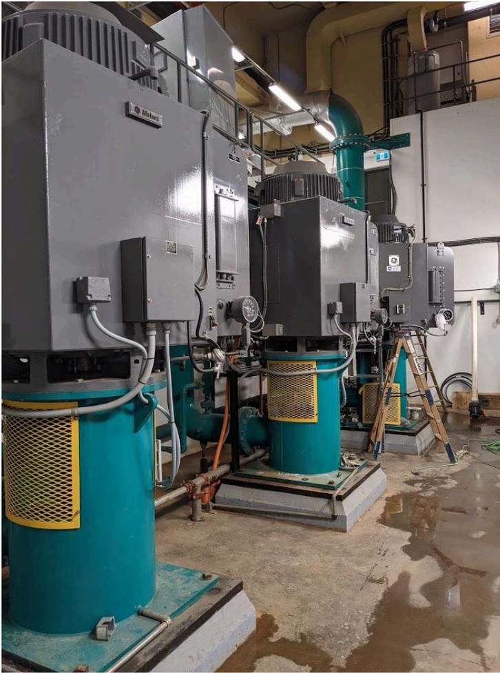
The Okanagan Lake Pumphouse is equipped with three 750HP high-capacity pumps, which are responsible for supplying water to the Okanagan Lake distribution system. This facility is the largest supplier of domestic water within our community, thus making it critical to ensure continued smooth operation.
